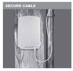
7b. Use the included zip ties and hardware to secure excess cable near the battery pack, leaving enough slack for a "drip-loop," preventing rain water from trailing into the battery pack, Installation is complete.
